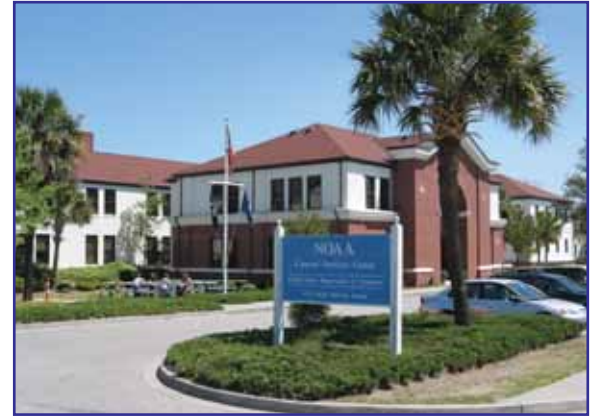
The NOAA Coastal Services Center in Charleston South Carolina.
