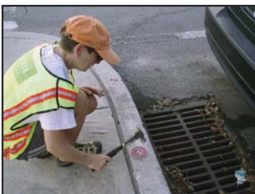
Anne Kitchell, volunteer project coordinator, demonstrates the installation of a storm drain marker in Beaufort, South Carolina. (Photo courtesy of SC NEMO.)
