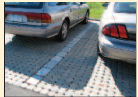
(Top) An example of a pervious parking lot located in Old Saybrook, Connecticut that can be found on the LID Atlas.
