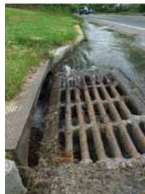
NY NEMO is helping Long Island Communities address Phase II stormwater issues.
