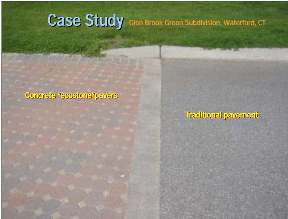
Lots of pictures in this presentation. Here's one from the Roads section showing pervious concrete pavers.
