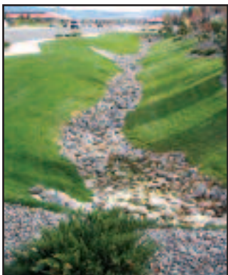
The city of Reno, Nevada is encouraging LID practices, such as this grass swale, to be used in all new development.
