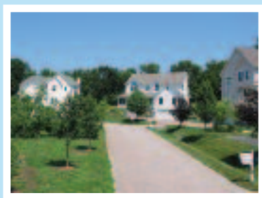
Individual homes at Jordan Cove have pervious driveway materials, rain gardens handling roof runoff, and “no mow” zones in the back yards featuring native vegetation. A sunken, vegetated cul-de-sac center accepts and treats runoff and there are swales located on each side of the street.
