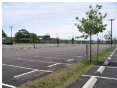
RI NEMO helped convince the University of Rhode Island to install two porous pavement parking lots.
