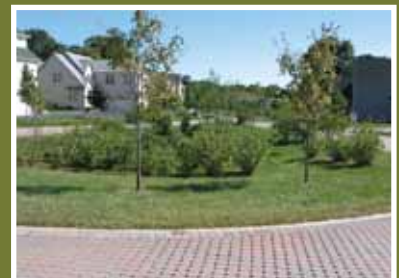
Sunken, vegetated cul-de-sac center accepts and treats runoff.
